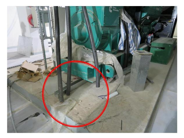
× Unavailable secondary power supply for FSIs and \_\_\_\_\_\_incomplete installation of emergency generator
