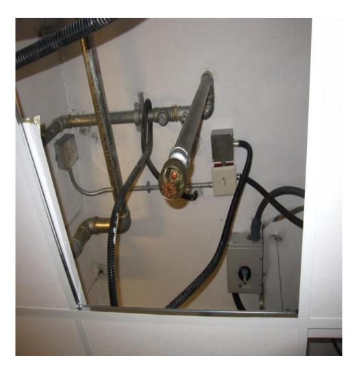
**x** Incomplete installation of concealed type sprinkler head
