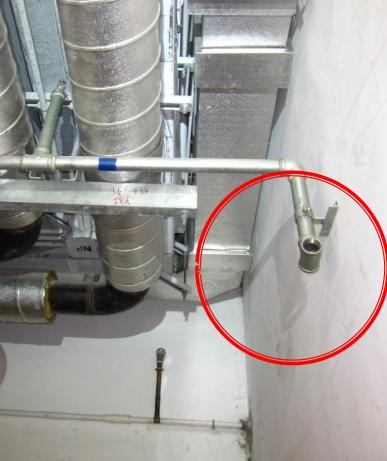
**x**Incomplete pipework of sprinkler system
