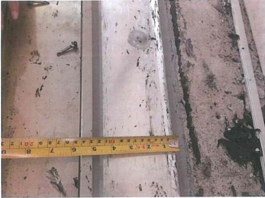
Photo 4: The static smoke barrier view from unexposed side
