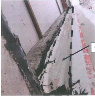
Photo 3: The static smoke barrier view from unexposed side
