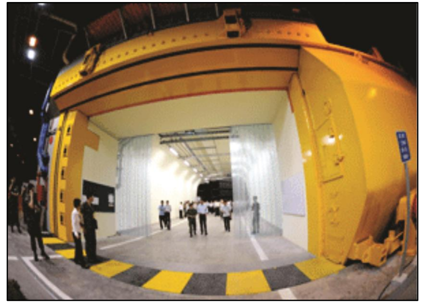
The Underground Ammunition Facility, Singapore
