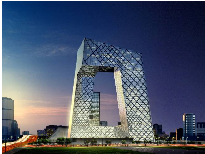
Figure 2: CCTV Main Building
