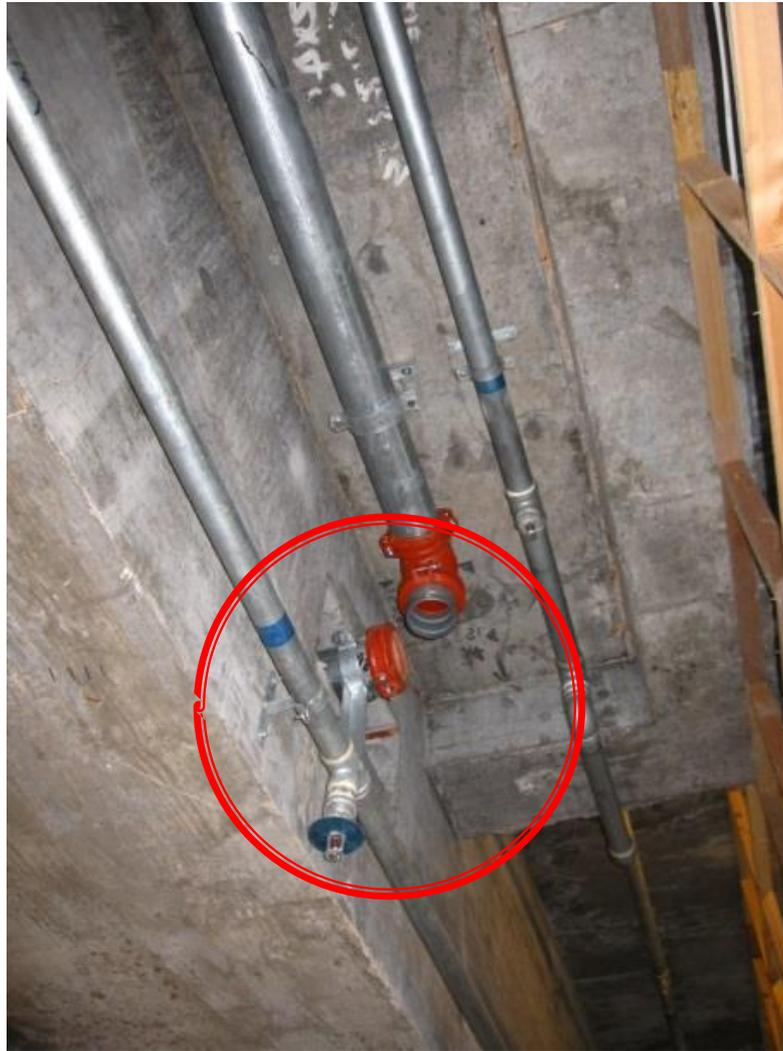
**x Incomplete pipework of sprinkler system**
