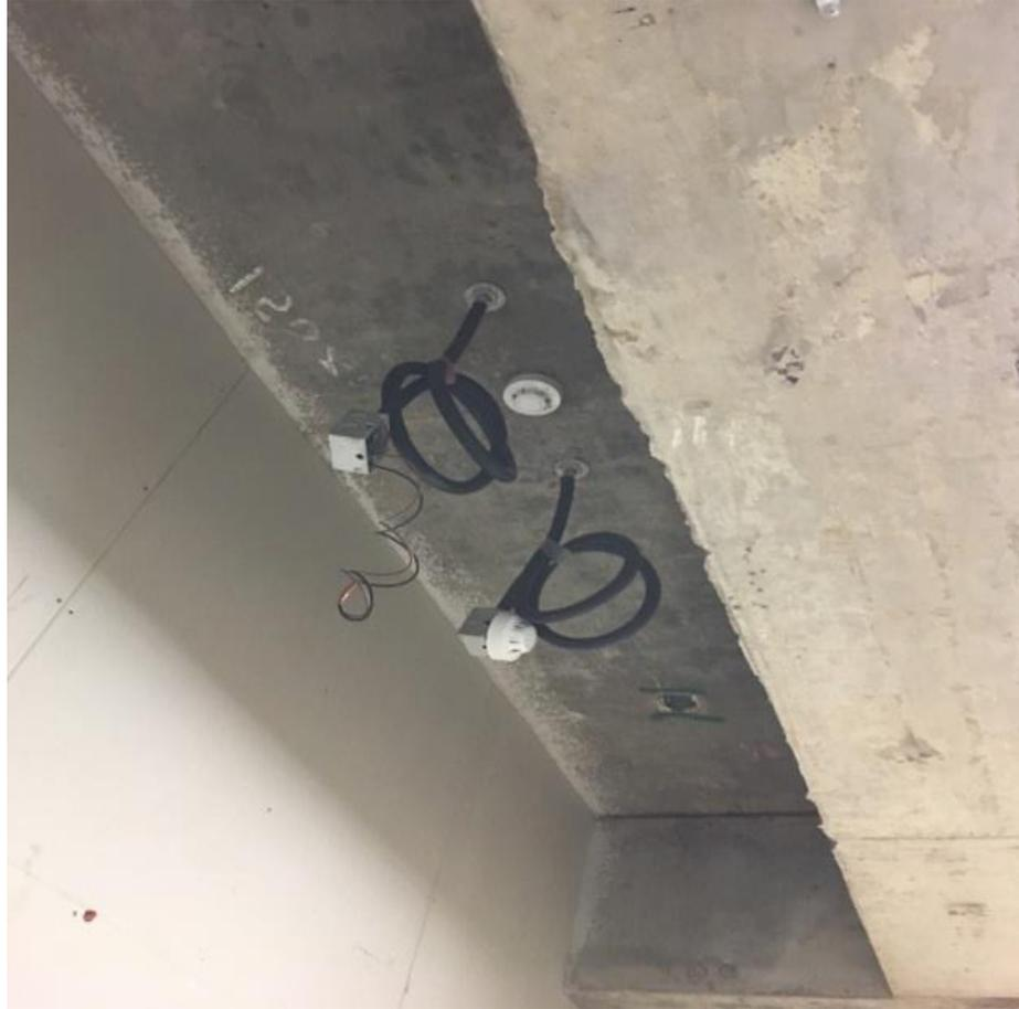
**x Incomplete installation of smoke detectors**
