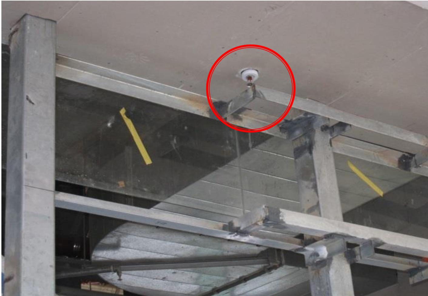
**x** Blockage of sprinkler head
