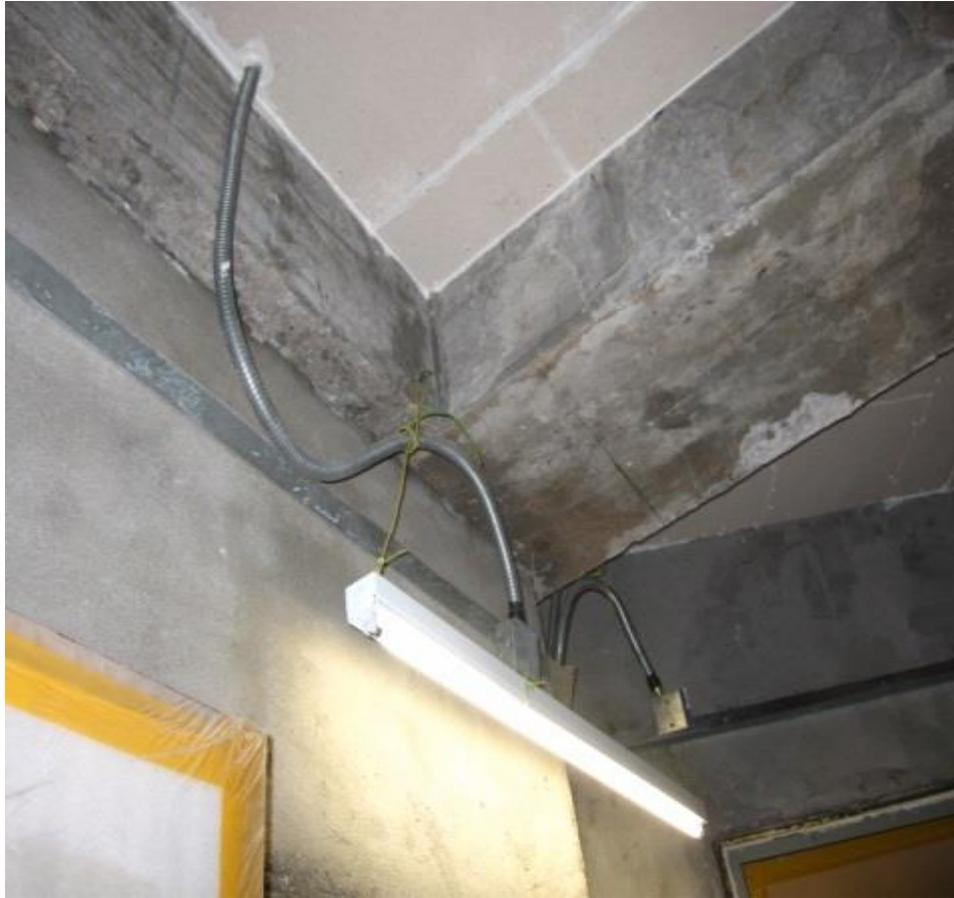
**x** Improper installation of emergency lighting
