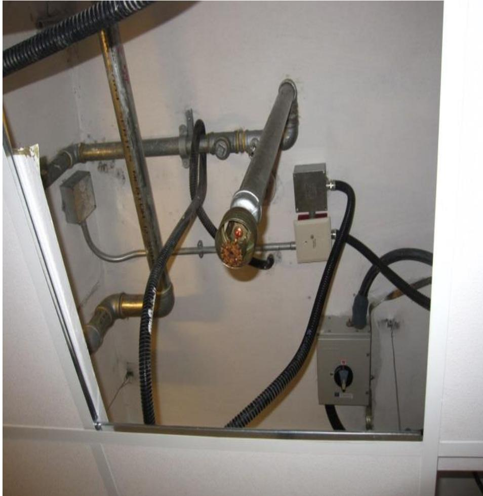
**x** Incomplete installation of concealed type sprinkler head
